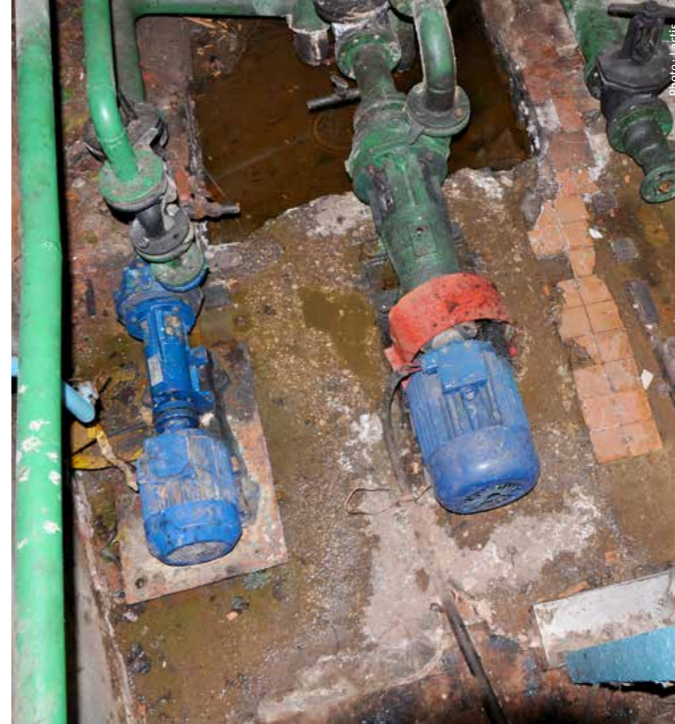
Electric motors were dismantled and operation was adjusted to the real pumping needs.
