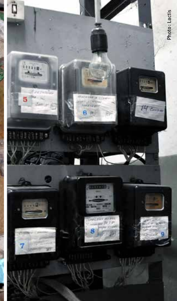
Old electric meters were installed to facilitate individual measurements.
